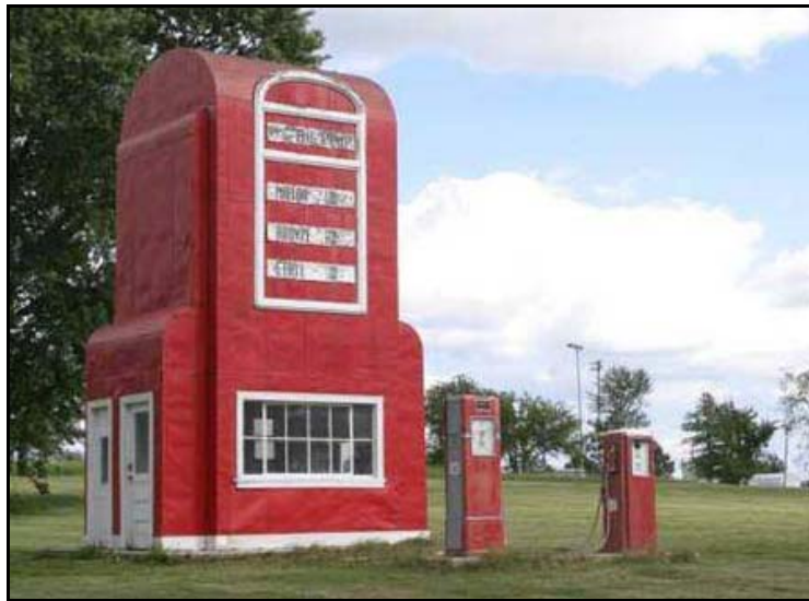
Old Gas Stations—No. 12 in a series
