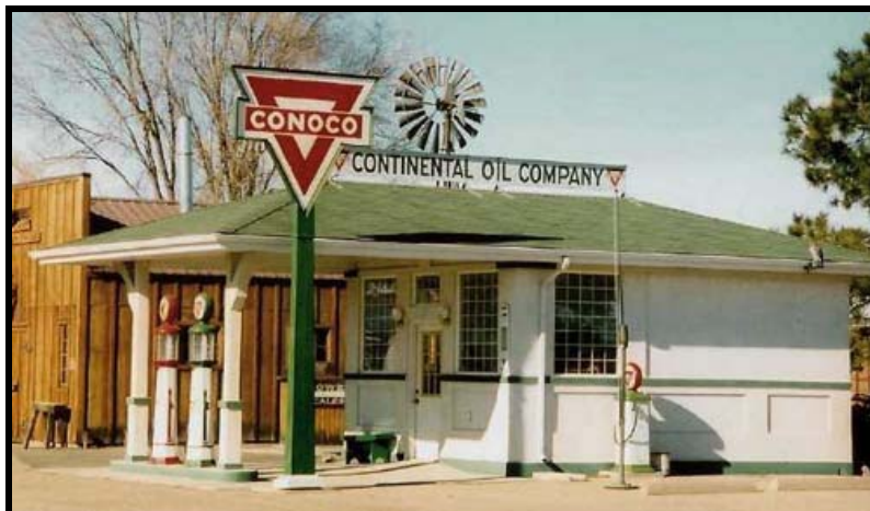
Old Gas Stations—No. 10 in a series
