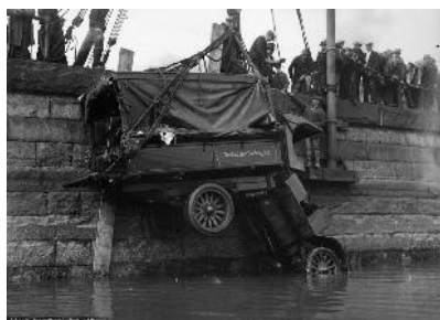
A Cudahy Packing Co. truck is hauled out of Fort Point Channel, which separates South Boston and downtown Boston.
